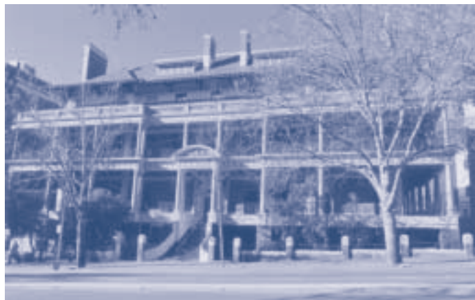
Margaret Graham Building, Royal Adelaide Hospital, South Australia
