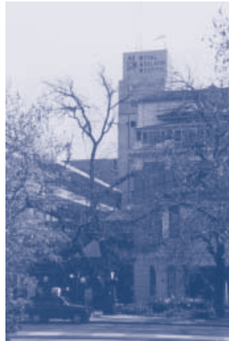
Royal Adelaide Hospital, South Australia
